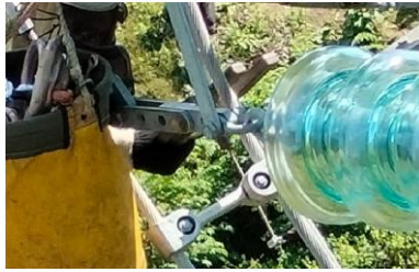
Figure 4. Installation of Ohm Stick Plus
