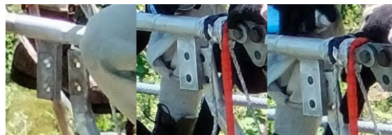
Figure 11. Cleaning Dirt from the Jumper Clamp
